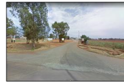
Transnet Tarlton Depot
