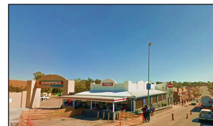
Wimpy at the southern entrance along the R24
