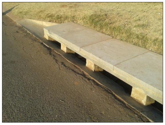
Cover slabs for Storm water catch pits : Various Types
